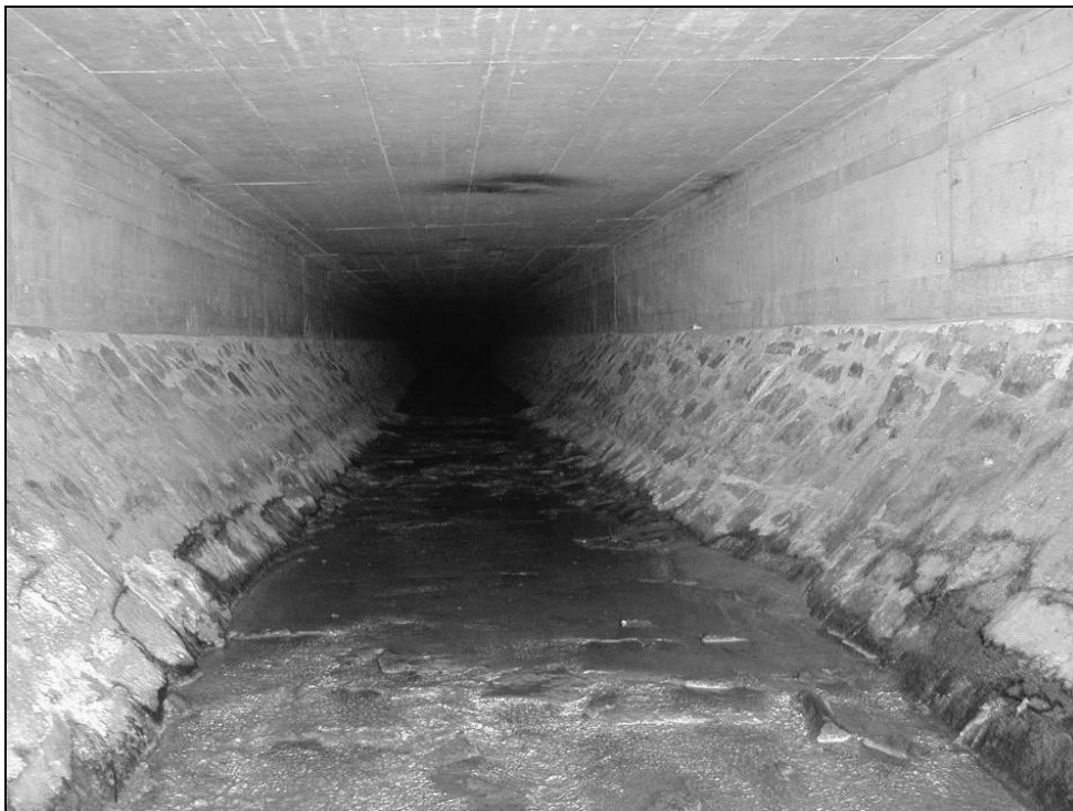
Figure 3: The Schweinbach Brook as an example for a tubed water course.
