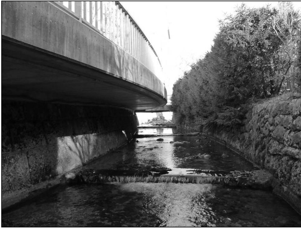
Figure 2: The Sulzbach Brook nearby Bad Ischl is an example for the missing longitudinal connectivity in water courses.
