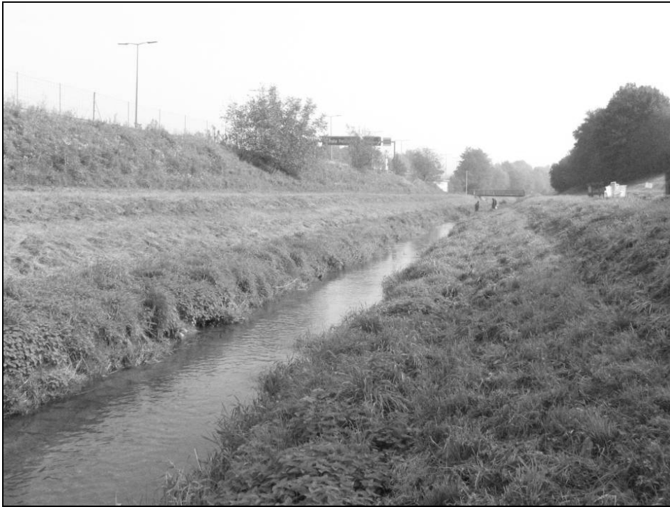
Figure 4: An artificial water course in Linz called “Urfahrner Sammelgerinne” before the restoration. The technical control structures that reach from the bed to the upper edge of the banks are not visible as they are covered with soil and vegetation.
