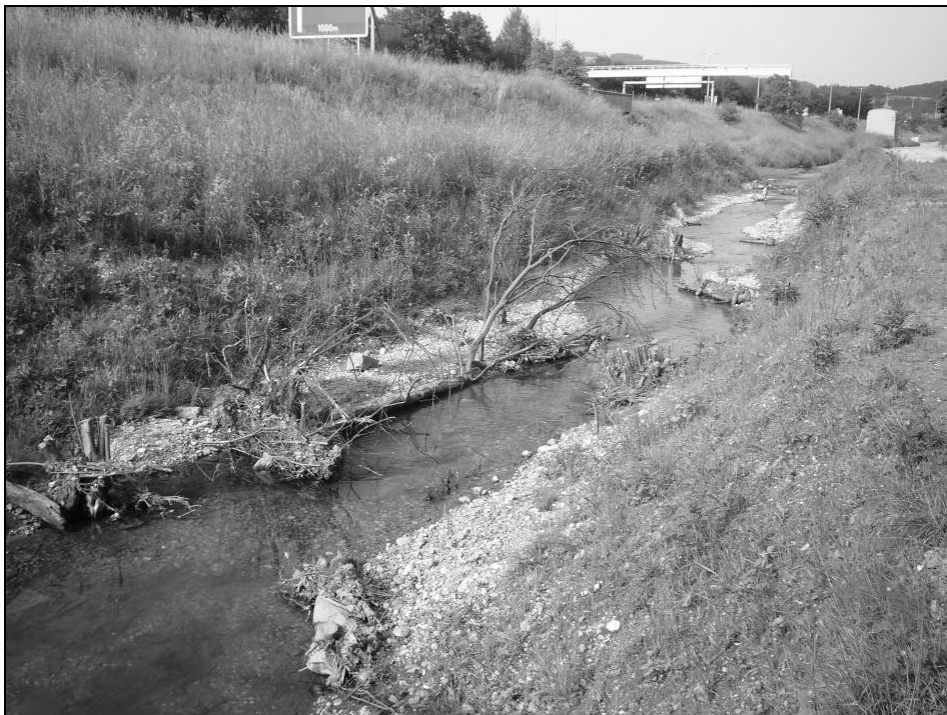
Figure 5: The “Urfahrner Sammelgerinne” in Linz after the restoration.
