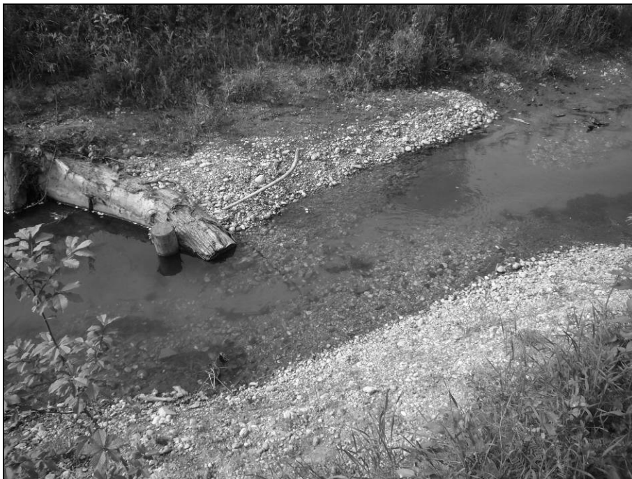
Figure 7: Nature-orientated bed of the “Urfahrner Sammelgerinne” in Linz after restoration.
